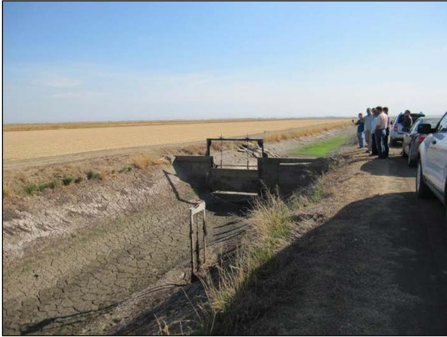
Figure 3. Existing Cottonwood Check Structure
